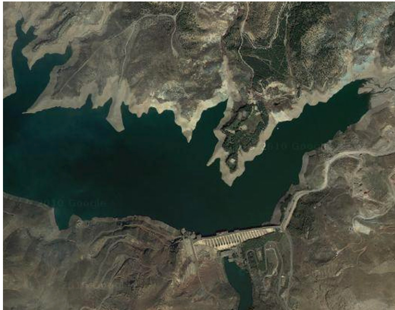
Fig. 9. Satellite image of Latyan dam and its reservoir.
